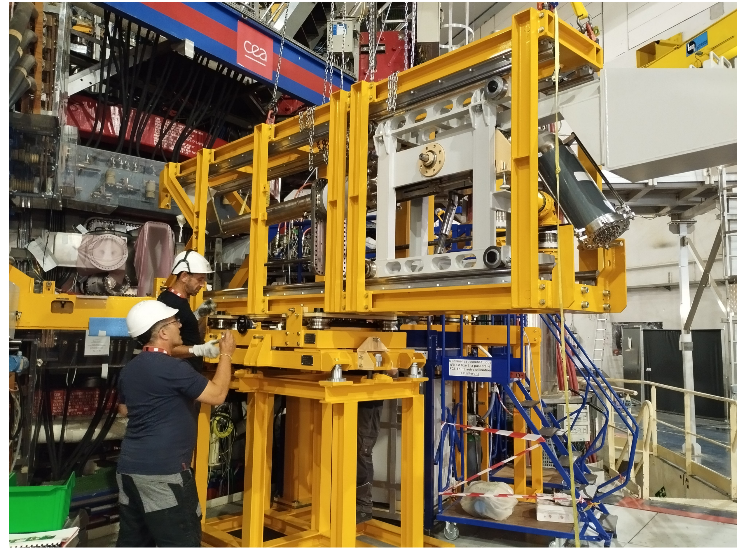
Fig 2. Installation of the Edge Diagnostic
