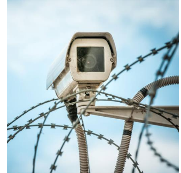
Credit: Nuclear Engineering International
