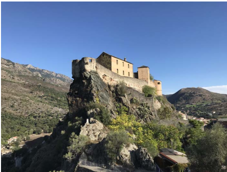
Fig. 10. View of the Corte castle (from South)
