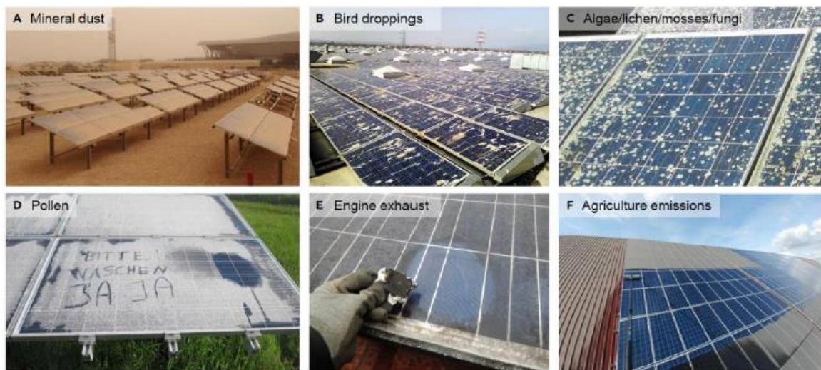
Figure 4: Example of (sources of) soiling in PV installations [2].
