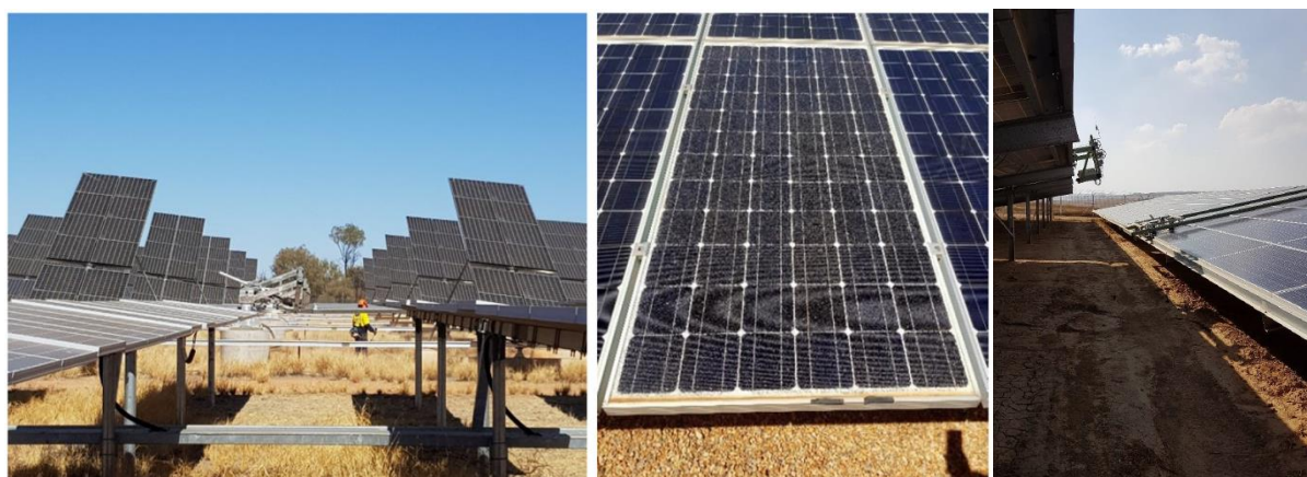
Figure 7: Left: Vegetation management of PV plant in Central Australia [2]; Middle: PV module (from a PV array in Central Australia) damaged during vegetation management due to pebbles [2]; Right: Automated cleaning of soiled PV modules in the Negev Desert, Israel [2].
