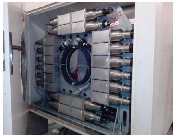
Fig. 6. Integration of C-BORD RRTNIS components in a temperature-controlled and sealed container (in view of further outdoor field tests) at CEA Saclay, France.
