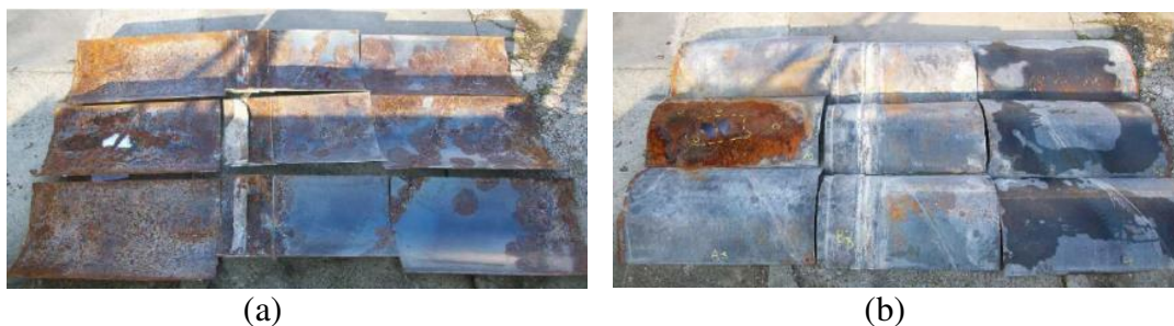
Figure 3: Pictures of corroded steel pieces, (a) inner side and (b) outer side
