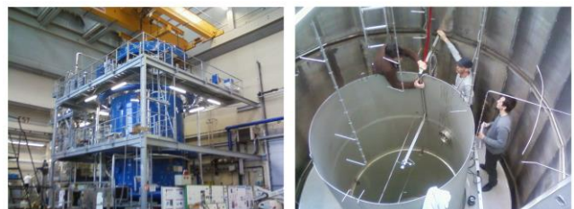
Fig. 9. View of the MISTRA facility (CEA Saclay) [21] (left) and installation of the probes inside the containment (right)
