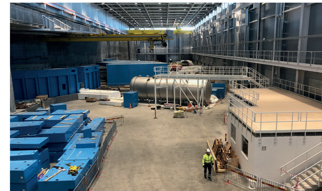
One of ESS’ instrument halls, showing the instrument, LoKI (a UK in-kind contribution), under construction. © ESS
