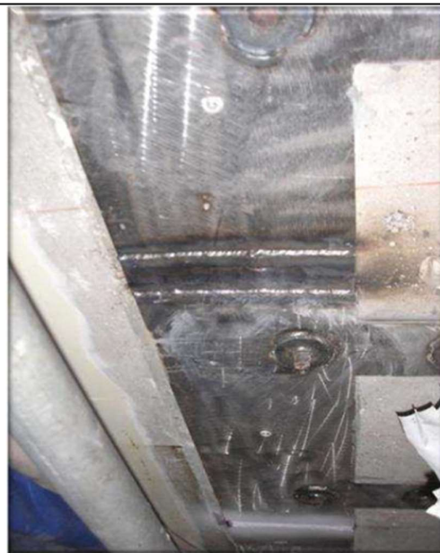
Bolting (embedding) and welding
