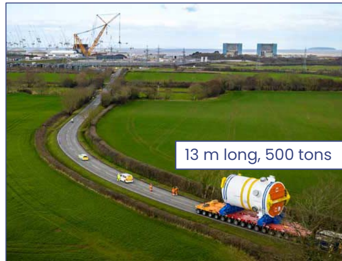
Hinkley Point C EPR reactor pressure vessel (UK)
