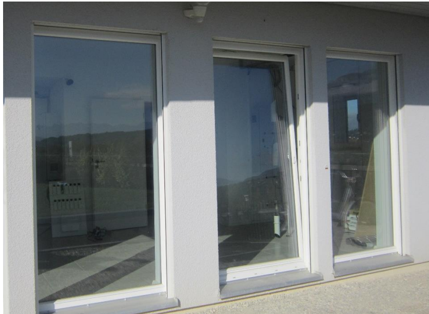
Figure 3: Tilt and turn window of woodframe House (L-B) South face, ground floor.
