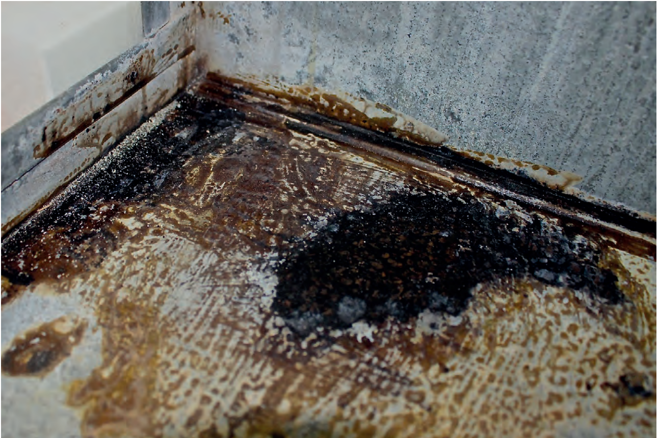
Figure 7 | Representative area of the brown/black crust on the bottom of the units. Photo by the author ©.
