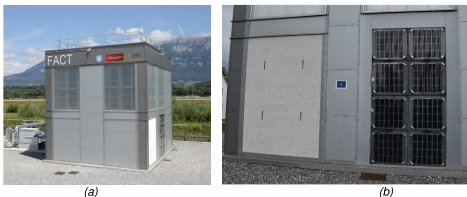
Figure 4: Photographs of FACT tool (a), of the south-oriented reference wall (on the left side) and of CONIPHER project BIPV wall (on the right side) (b) at CEA site (at Le Bourget du Lac)
