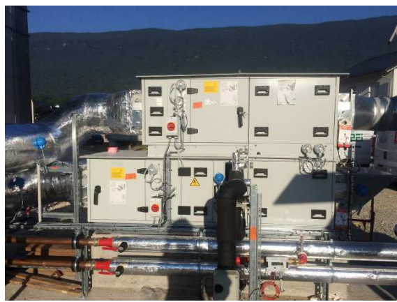
Figure 5: Location of the test cell 3 and the test cell 4 on a plan of FACT tool ground floor (a) and dual-flow air handling unit (CIAT) (b)
