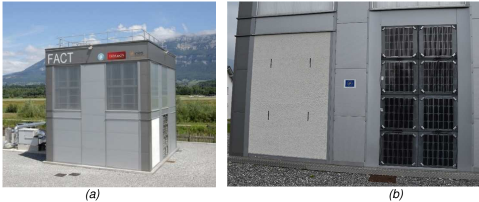
261 Figure 4: Photographs of FACT tool (a), of the south -oriented reference wall (on the left side) and of CONIPHER 262 project BIPV wall (on the right side) (b) at CEA site (at Le Bourget du Lac)
