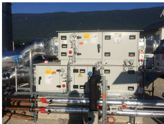
Figure 5: Location of the test cell 3 and the test cell 4 on a plan of FACT tool ground floor (a) and dual-flow air handling unit (CIAT) (b)
