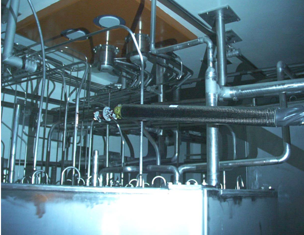
Fig. 21- Inspection of a pipe
