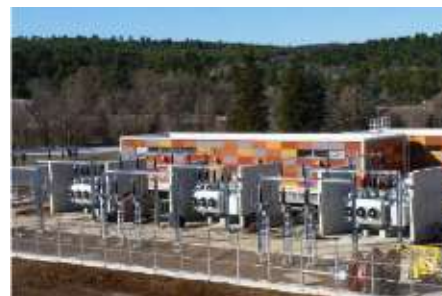
63kV / 15kV substation
