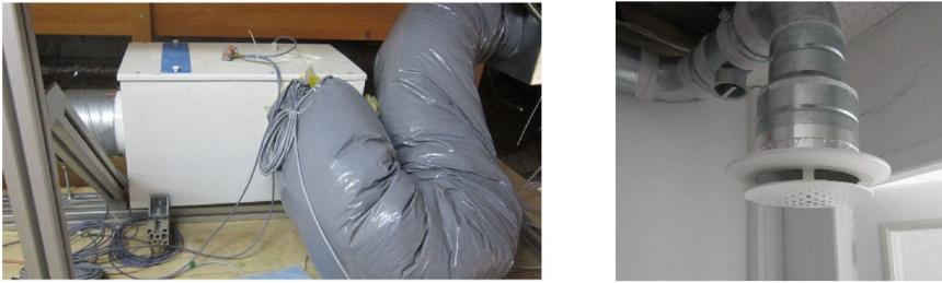
**Figure 1.** Pictures of the Positive Input Ventilation in the experimental house – Left: Central ventilation device in the attic, Right: Air diffuser in the first floor hall.
