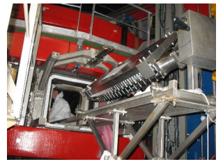
Removal of Q6A out of the vessel
