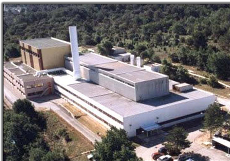
Fig. 1: The LECA STAR building
