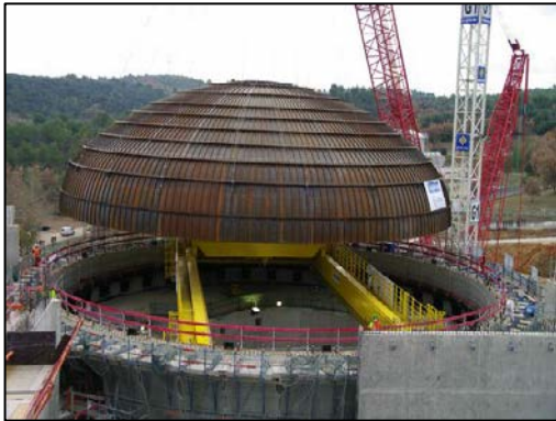
December 2013: Reactor dome installation © CEA
