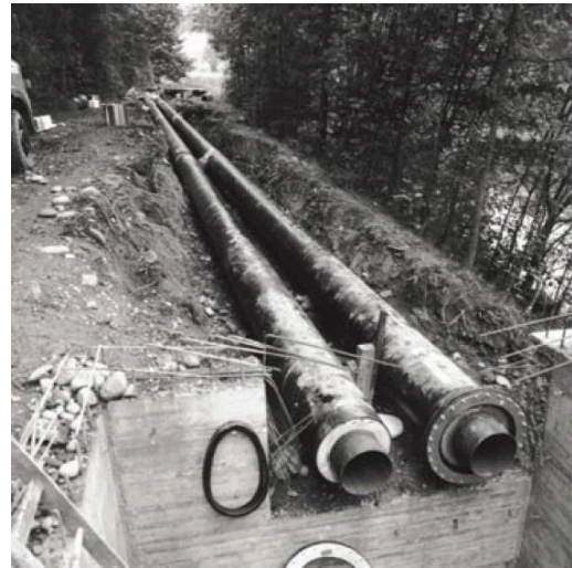
Fig. 1. Building the main heat transport line ([8])
