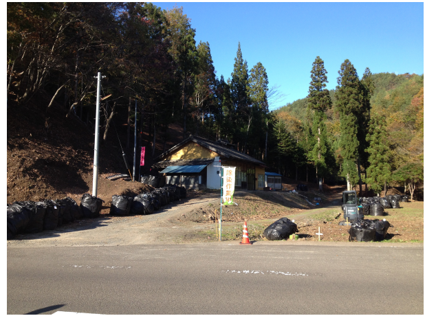
Figure 4. Illustration of the 20 m decontaminated buffer zone in forested areas in the vicinity of houses. Example from Iitate village (Sasu district).
