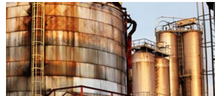
Atmospheric corrosion in a chemical plant
