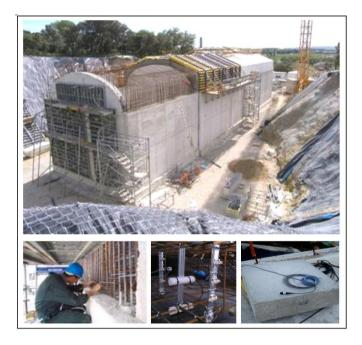
**Figure 9 :** Overall view during construction of the vault of GALATEE. View of the instrumentation embedded and of the comparison wall built during construction
