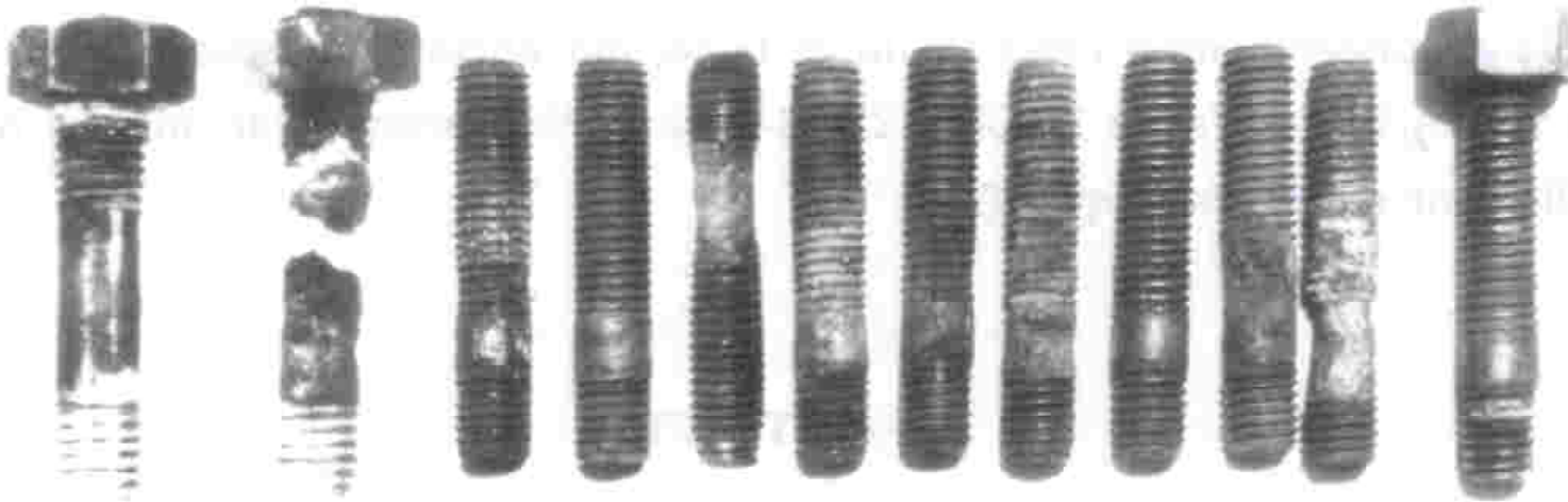
Bolts corroded by boric acid
