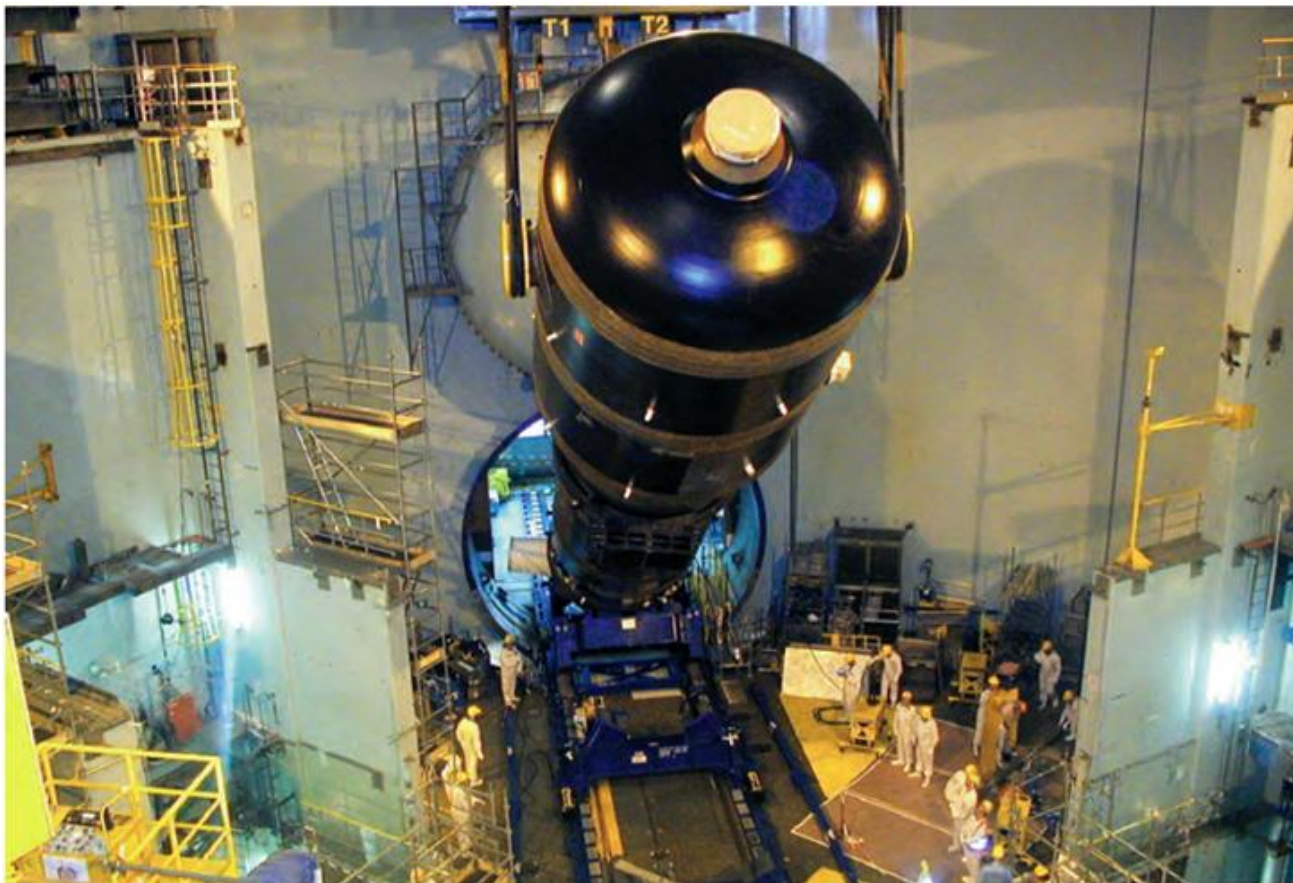
Replacement of a Steam Generator
