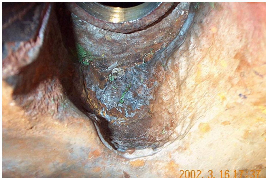
Nozzle 3 with insulation removed and shielding installed 03-16-02
