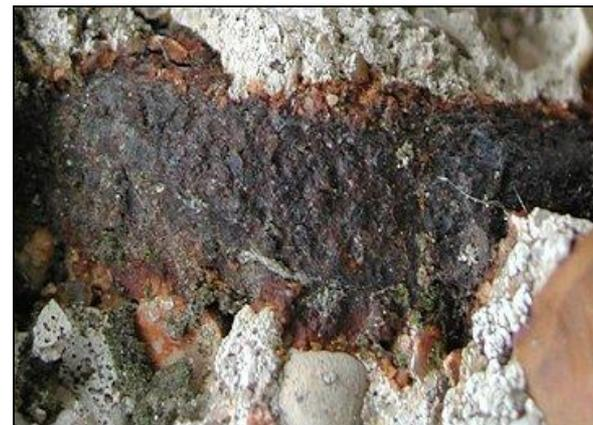
**Corroded steel rebars in concrete structure**
