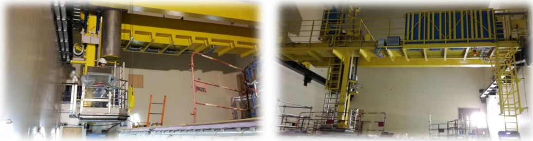
Fig. 6: One-site pool crane commissioning tests
