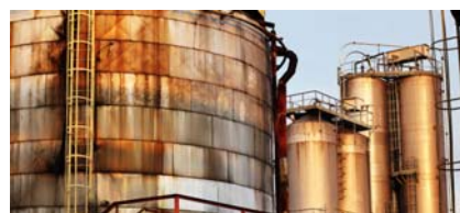
Atmospheric corrosion in a chemical plant
