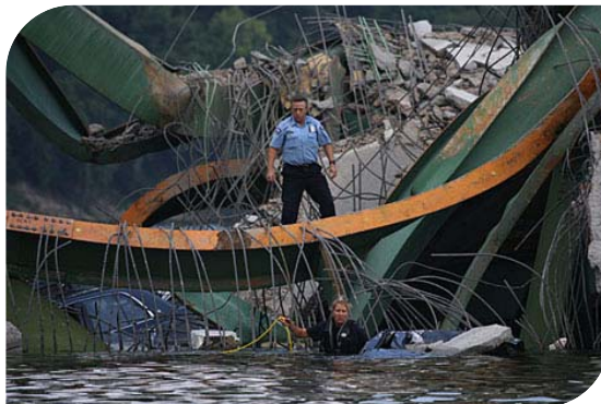
Mississippi Bridge, Minneapolis, August 1, 2007, 13 fatal structural weakness caused by corrosion
