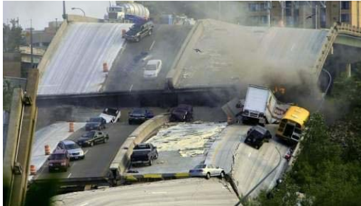
Highway bridge over the Mississippi, Minnesota, 2007 (40 years old, corrosion)
