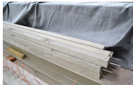
(b) Prismatic specimens intended to be corroded
