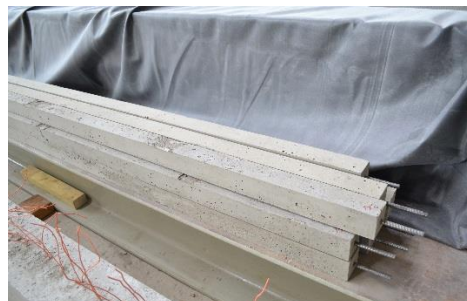
(b) Prismatic specimens intended to be corroded
