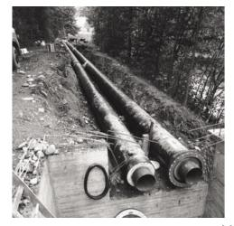
Fig. 1. Building the main heat transport line [9].
