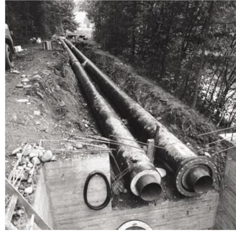
Fig. 1. Building the main heat transport line [9].
