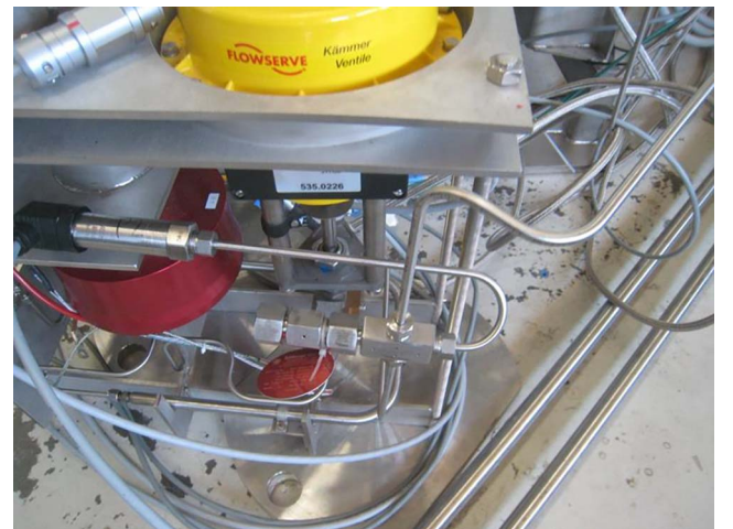
Fig. 3. View of the throttle valve in the MEXIICO installation.
