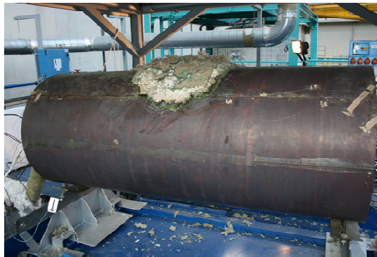
Figure 4. FUTUNA mock-up pipe after the leakage experiment (on top, the heat insulator burned by the liquid sodium)
