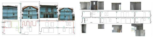
Figure 3. Optical fiber cables routing under the thermal insulation of external walls of house BB (left), Fiber routing under the house BB internal walls decoration (right).
