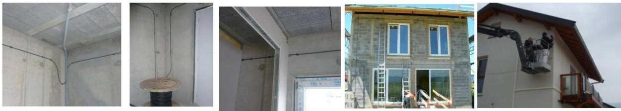
Figure 5. Routing at room corners. Cable drum. Routing through an internal wall, Deployment on external surface.
