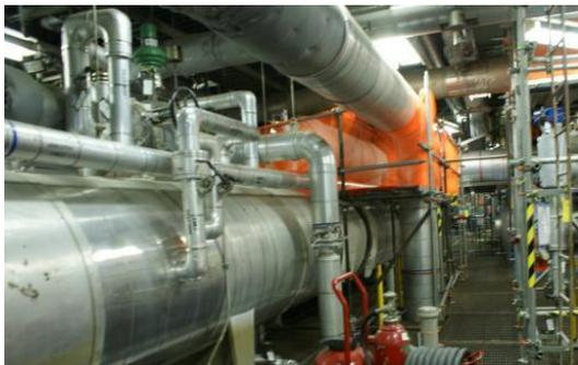
Fig. 3 Example of steam pipes able to be monitored with optical fibers for distributed leakage detection.
