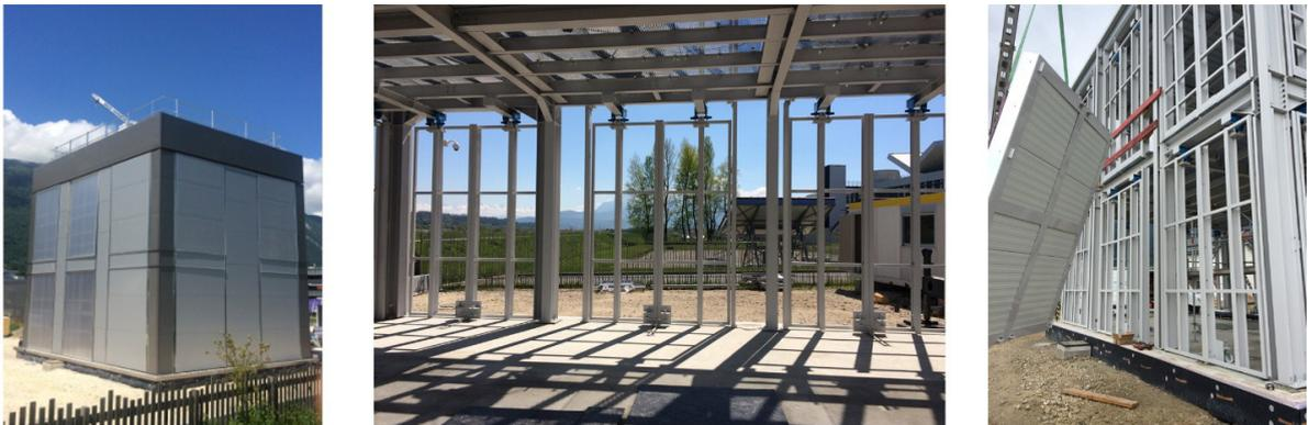
Fig. 3. FACT during the building phase. External view (left), the secondary structure (center) and façade installation (right).
