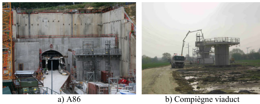
Figure 1. General view of the construction sites.
