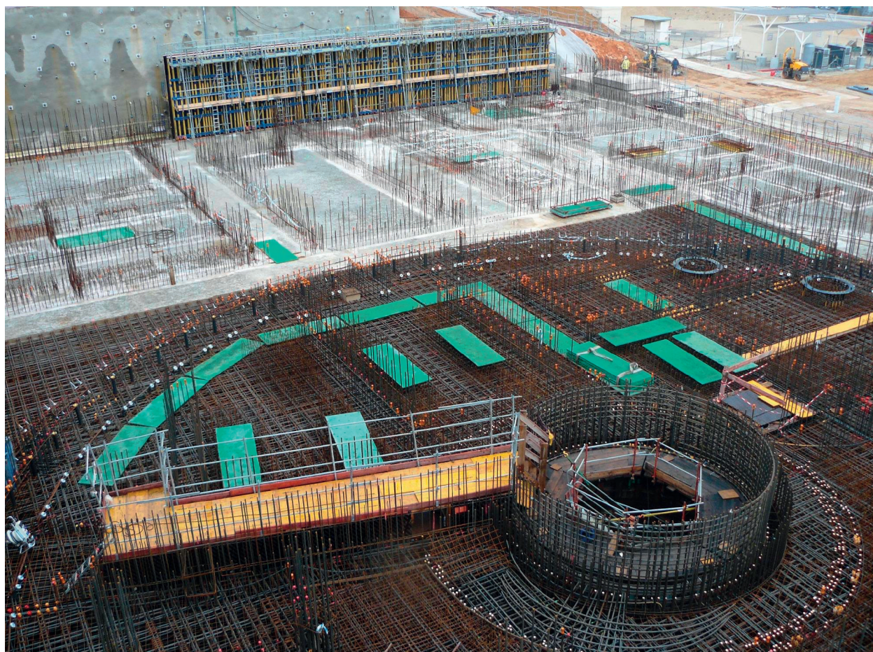
Fig. 96. The Jules Horowitz Reactor construction site at CEA/Cadarache site (March 2011).
