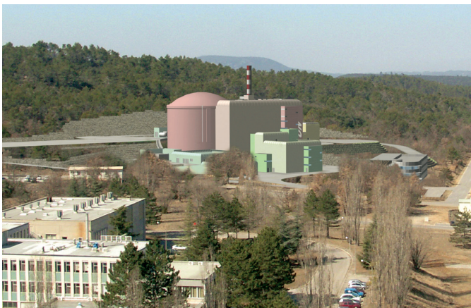
Fig. 91. Artist's view of the Jules Horowitz Reactor Project at the Cadarache site.
