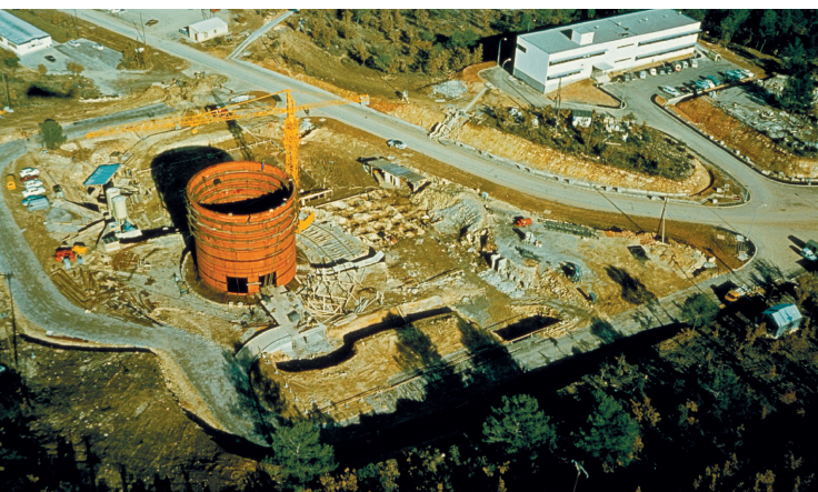
Fig. 47. Construction of the MASURCA reactor.
