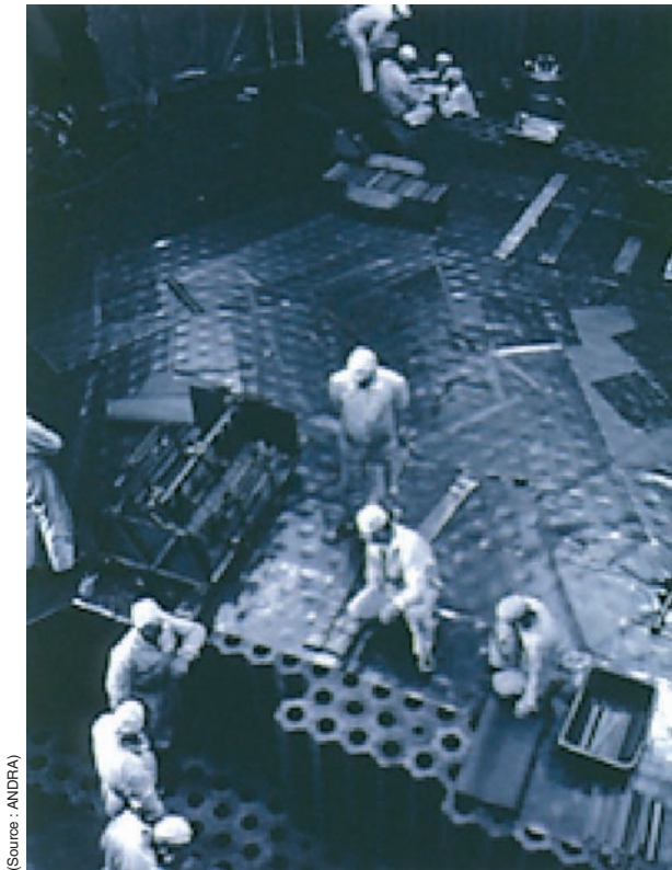
Fig. 54. View of the graphite block pile in the Chinon NUGG reactor.
