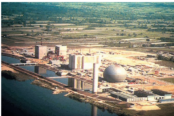
Fig. 9. The NUGG plant in Chinon.
