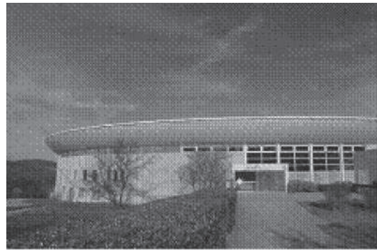
Fig. 9 INSTN training center in Cadarache (France)
