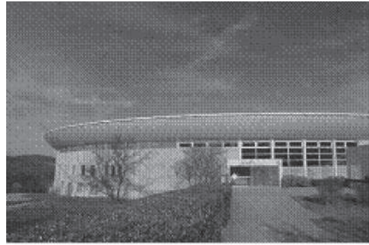
Fig. 9 INSTN training center in Cadarache (France)
